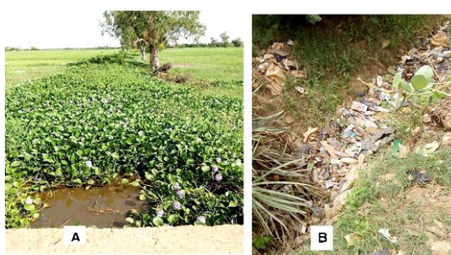
Figure 3: Grassing of canals and drains in wet season at Kirkissoye (A: main drain and B: secondary canal).
