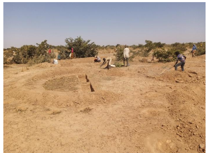
Fig. 5: Construction of anti-erosion works (multifunctional half-moon) on a degraded site
