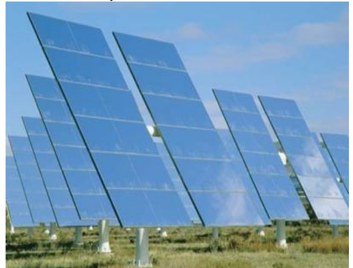
An Array of Solar Panels.
