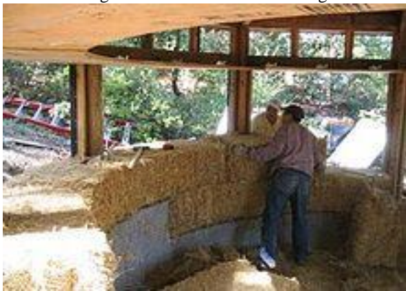
Walls Constructed with Straw
