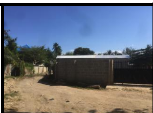
Figure 26: Mzee Mwaipaja Residence Source: Author, 2016
