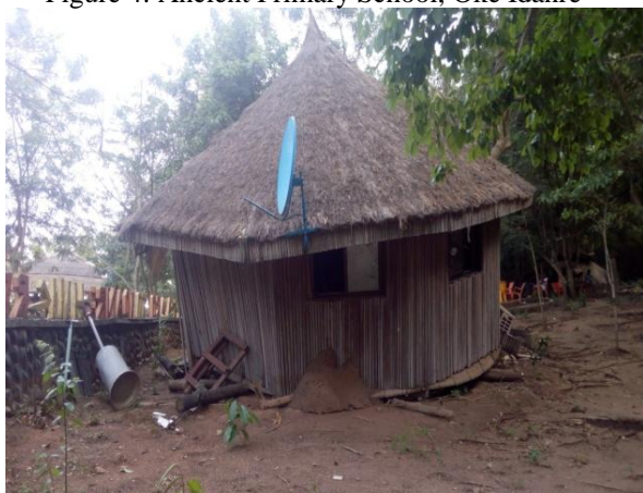
Figure 5: Dilapidated Tree House constructed by Dr. Mimiko administration at Oke Idanre.
