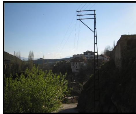
Figure 7 One of the electric poles in the city.
